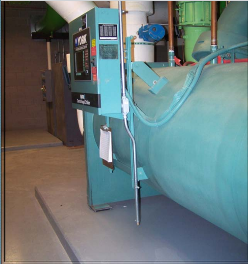
New Supported Installation
